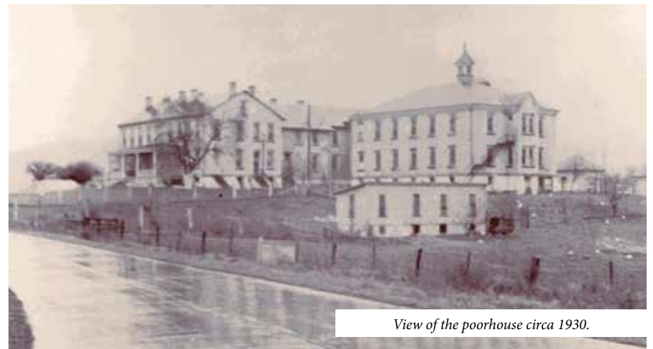
The poorhouse is now the GCHS Museum.
